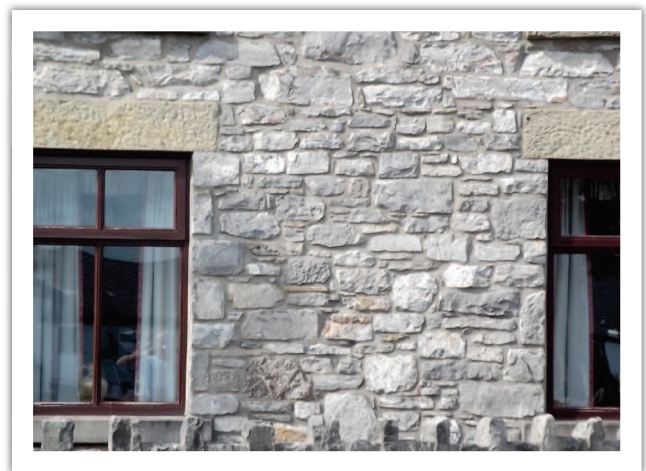
» Structural stone walling is coursed to ensure it will hold up on its own. Stone lintels support the structure over the doors and windows
