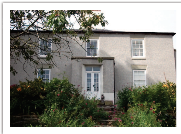
» Although much altered, the Old Vicarage still has sliding sash windows of the type many houses in the village from the late Georgian and Victorian period would have had.
