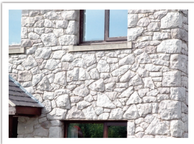
» Modern construction uses stone only as a cladding material and it can appear to lack strength or purpose
